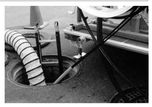
**Figure 7-7** Two fiber optic cables being pulled through innerduct that has previously been pulled into conduit. Courtesy Condux
