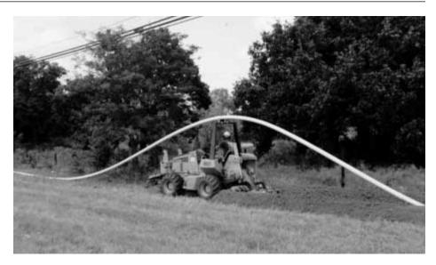
**Figure 15-1** Fiber optic cable is often installed in conduit for outside plant applications.
